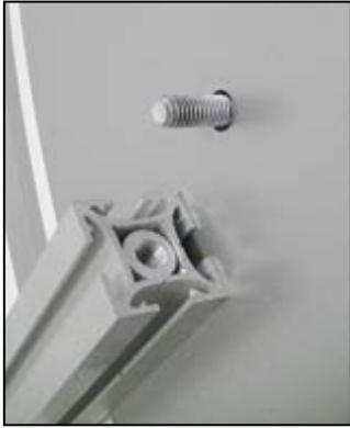
Base Plate Connection
